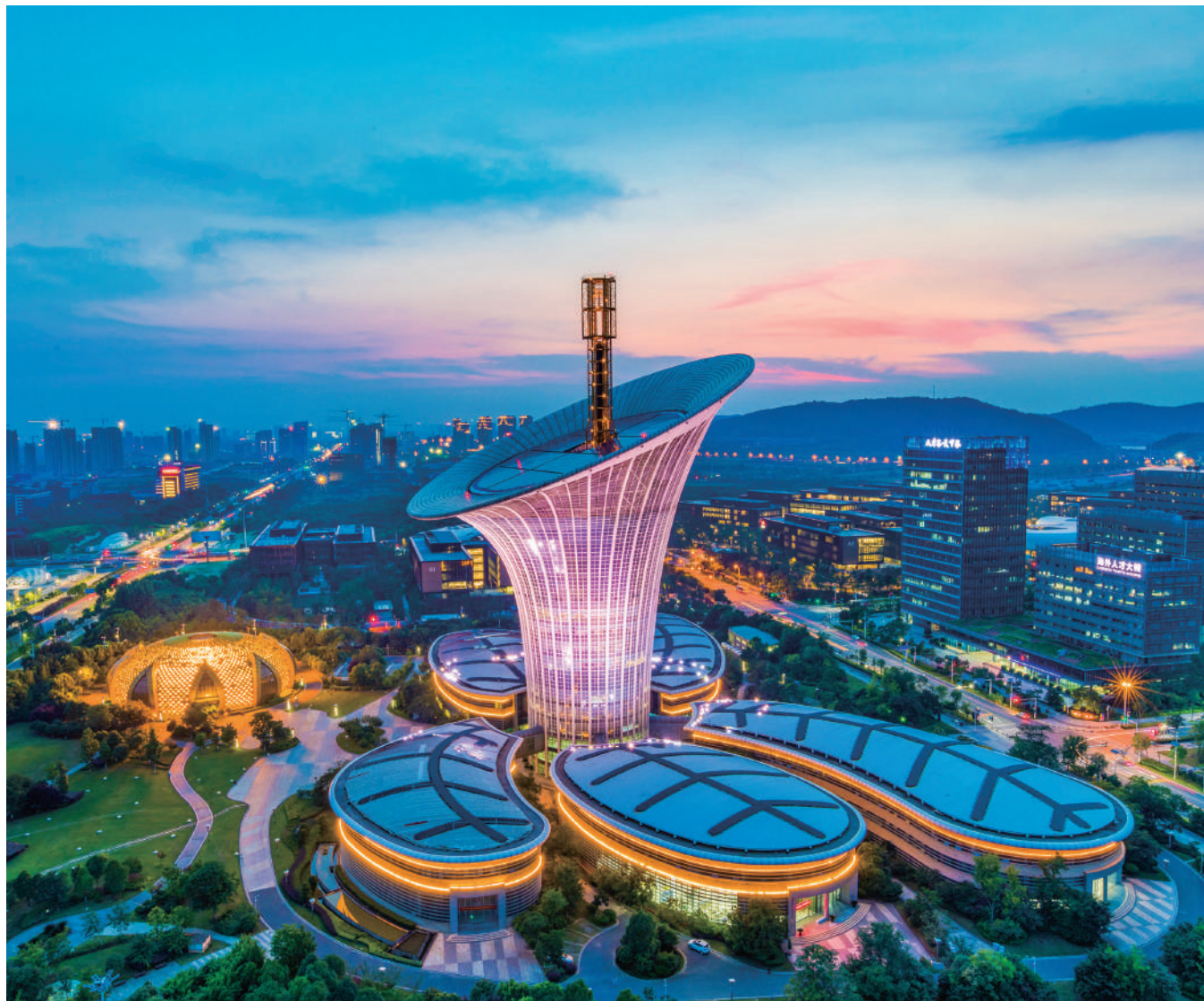
Future Technology City at Wuhan Optics Valley (Photo by Jiang Tao)
